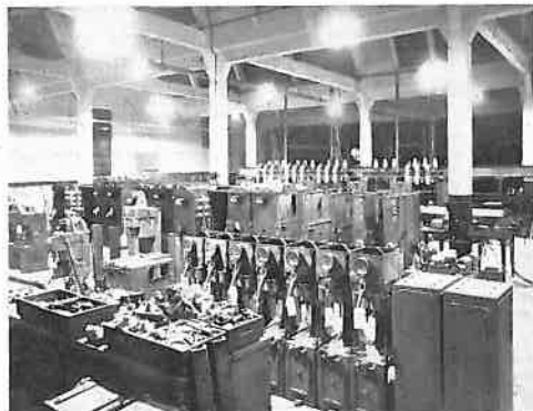
Heavy Assembly Room.
