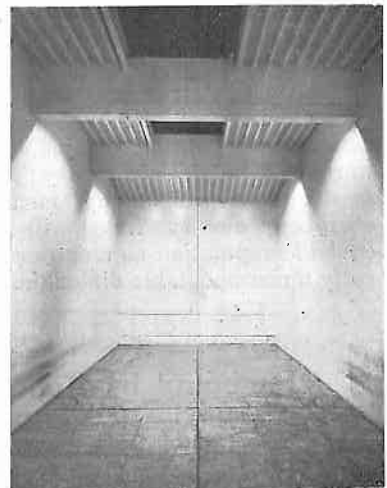
Night photograph of Squash Racket Court lighted by Mazda lamps in X-ray reflectors.
